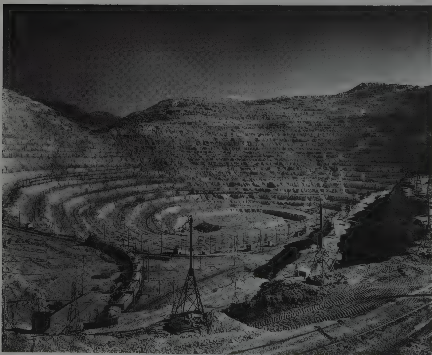
28 The Bingham copper mine near Salt Lake City is the largest surface copper mine in North America. It covers 1,050 acres and contains about 175 miles of railroad track. After the copper has been mined what might be done with the excavation? ( The Bettmann Archive )
