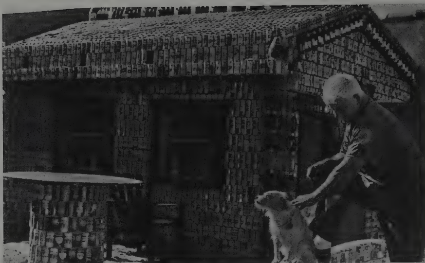
22 Examples of houses made from waste materials are found in most countries. This one was made of cans and bottles on a steel frame by Walter Sizemore in San Jose, California. ( East San Jose Sun )
