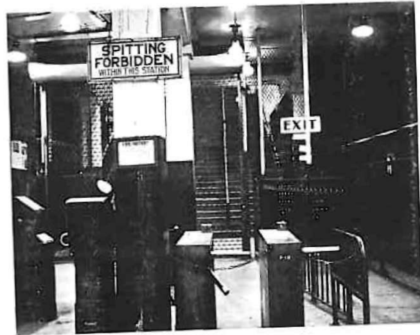
FIG. 29. The nether world of the subway
